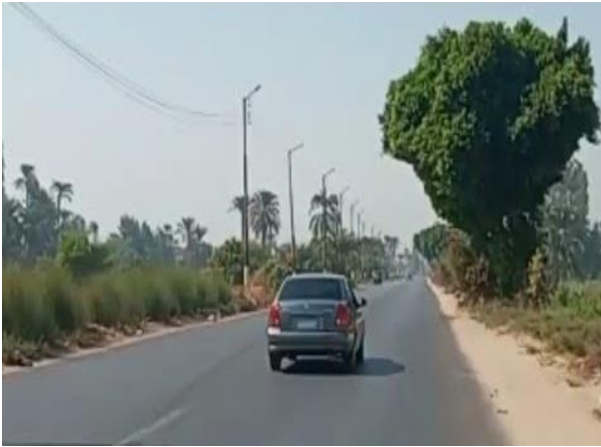
Figure 9 photo of Egypt Rural Road
